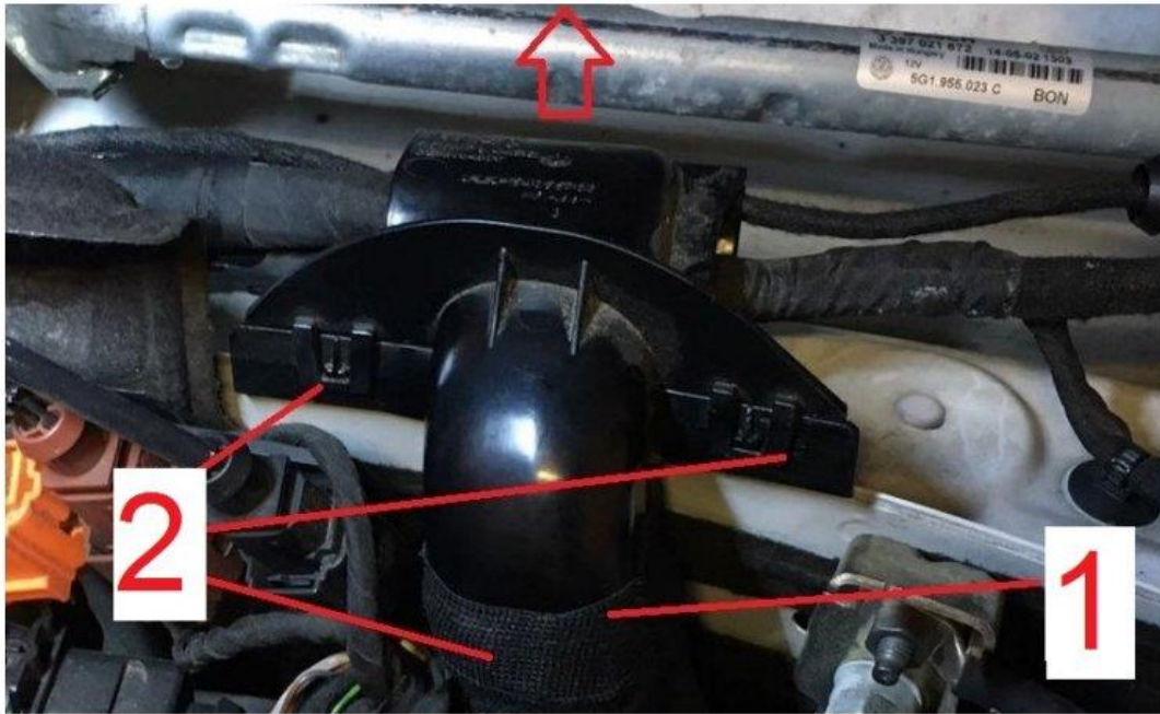
Prepare cable routing
